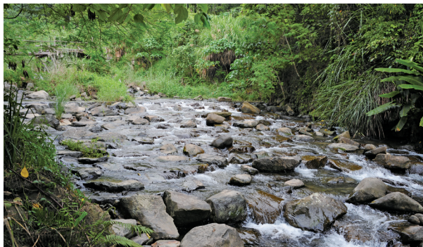
▲ The fifth construction of the improvement for Duen-abanang stream in Alishan Township, Chiayi County
